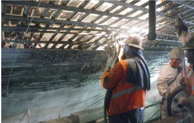
Fig. 7: Nozzle in outer layer of reinforcement, encasing the back layer
