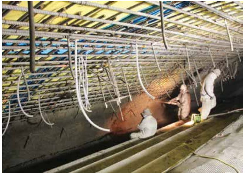
Fig. 2: Overhead arch—lower panel being built up. Note the BA anchors and injection tubes displaying the depth of the concrete section
