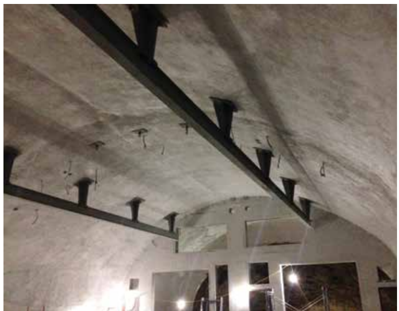
Fig. 4: Final arch structure shotcreted in layers due to thickness
