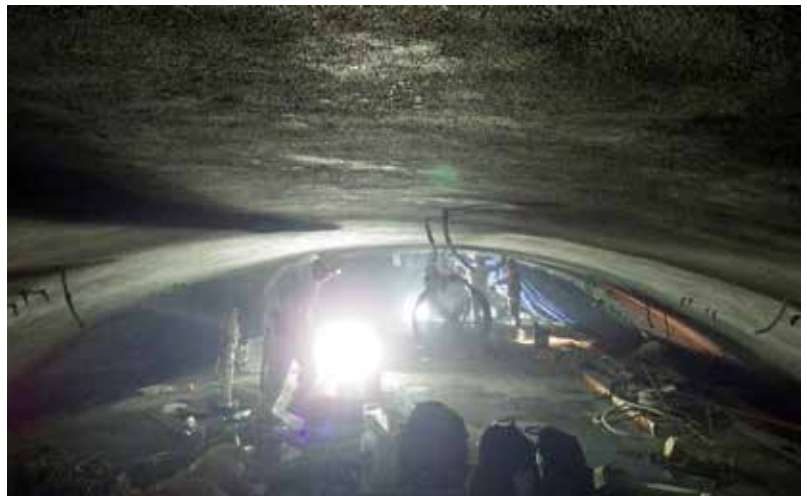
Fig. 3: Working on final panel—heat presented a challenge, requiring ventilation and close attention to curing
