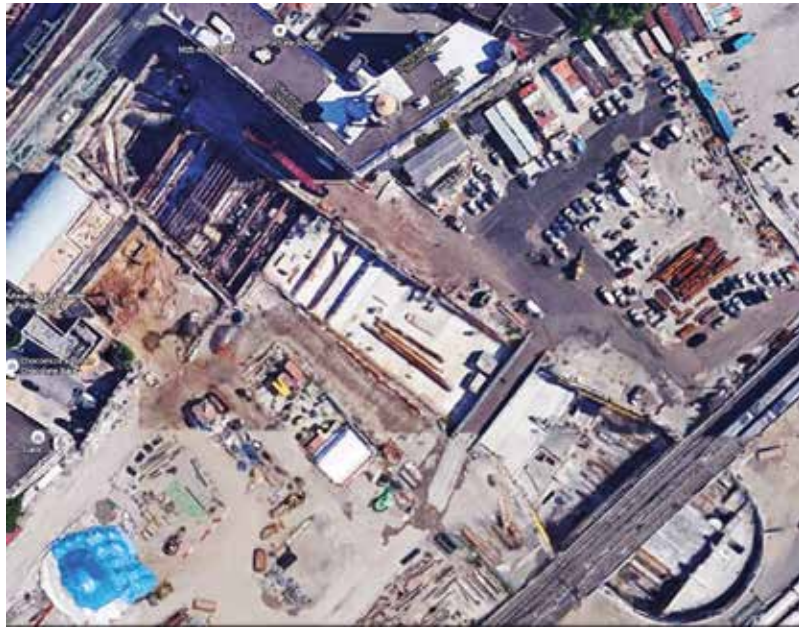
Fig. 1: CQ32 is a four-level ventilation facility, passenger station, and office for the MTA. Five other active projects are adjacent to and/or tie directly into the project, making logistics a challenge
