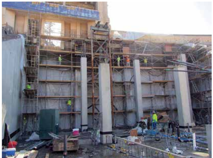
Fig. 4: Existing historic wall prior to shotcrete overlay application
