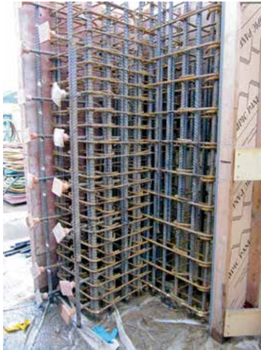
Fig. 2: Type 1 preconstruction test panel was composed of three curtains of No. 10 (No. 32M) and No. 9 (No. 29M) reinforcing steel with additional boundary reinforcing bar elements
