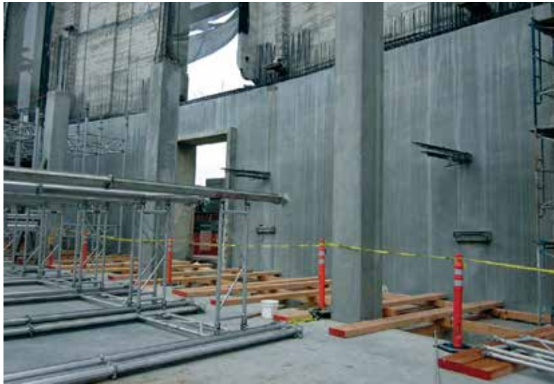
Fig. 6: Existing historic wall after shotcrete overlay application
