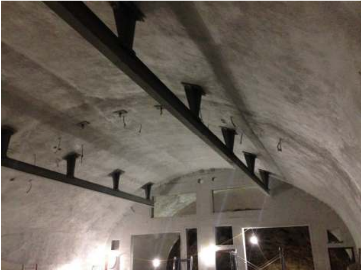
Final arch structure performed in layers due to thickness
