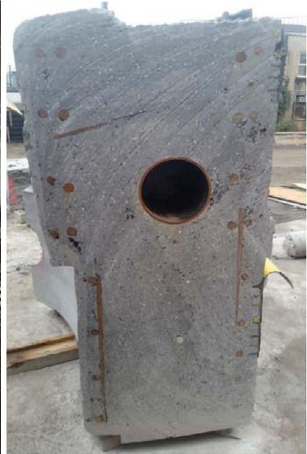
Encapsulation around reinforcement and embedments, and encasement of water barriers.
