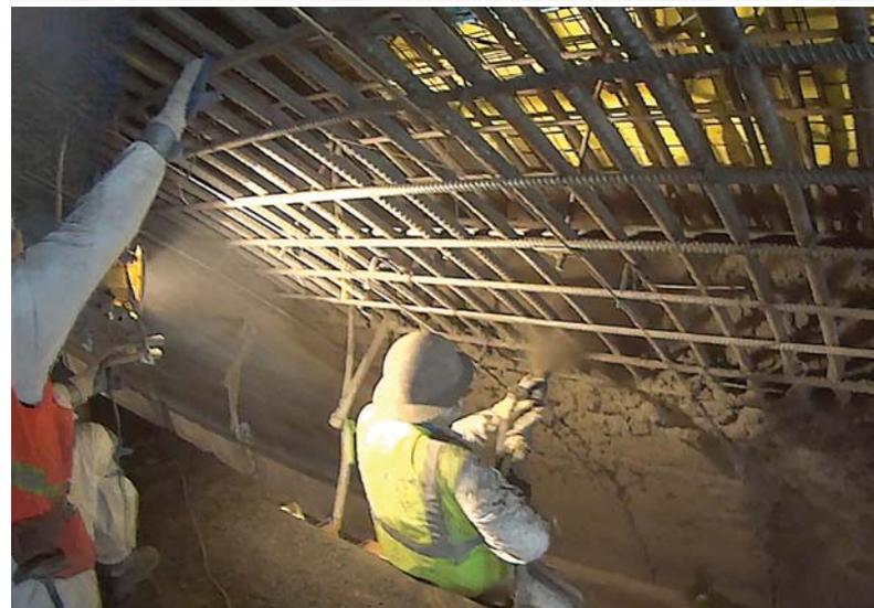
Using PAC for different applications – 30-inch-thick (762mm), 60ft-wide (18m) sequential excavation method (SEM) tunnel constructed through frozen ground.
